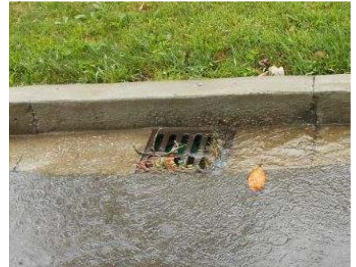
Next inlet downstream
