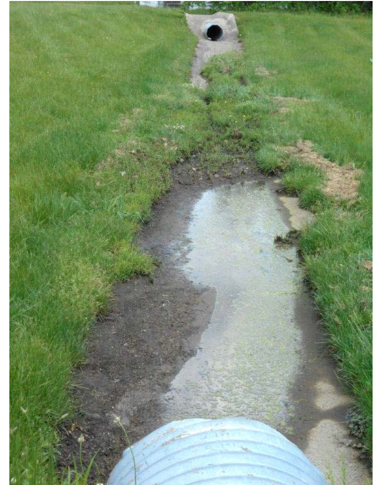
Downstream detention basin: future retrofit to improve WQ
