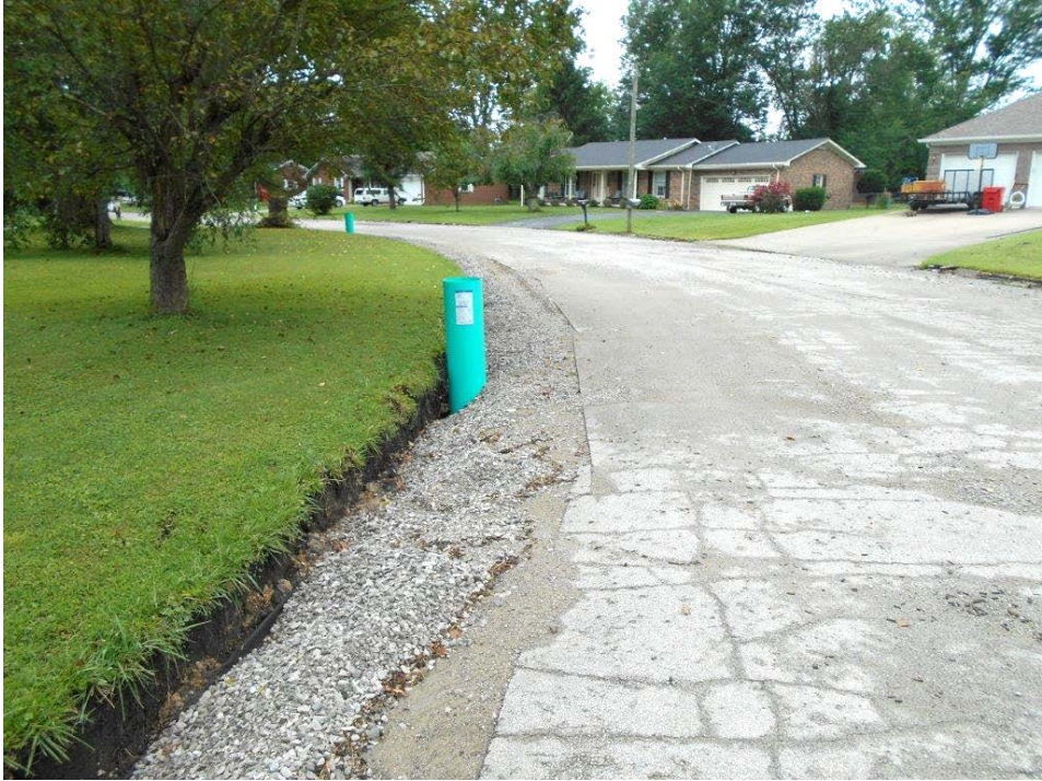
Detail "A" – replace curb & gutter
