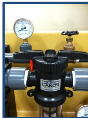
Manual Flush Filter
