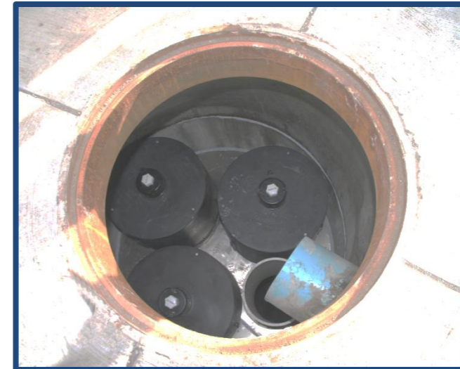
Manhole StormFilter
