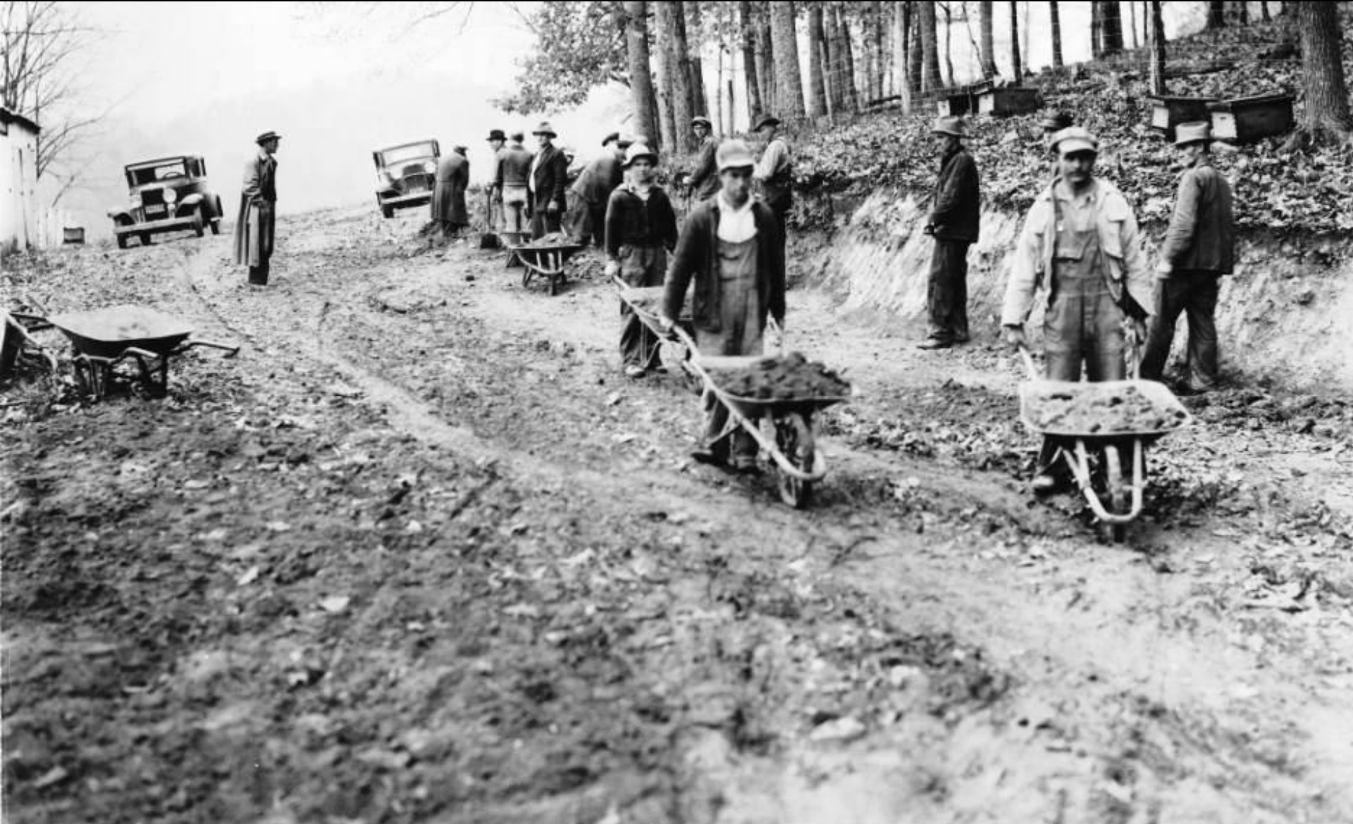
3095 Lock and Dam No 6, Green River E.R.A. Project OP 13-279 Men grading road at entrance to Government Reservation Oct 23-1931
