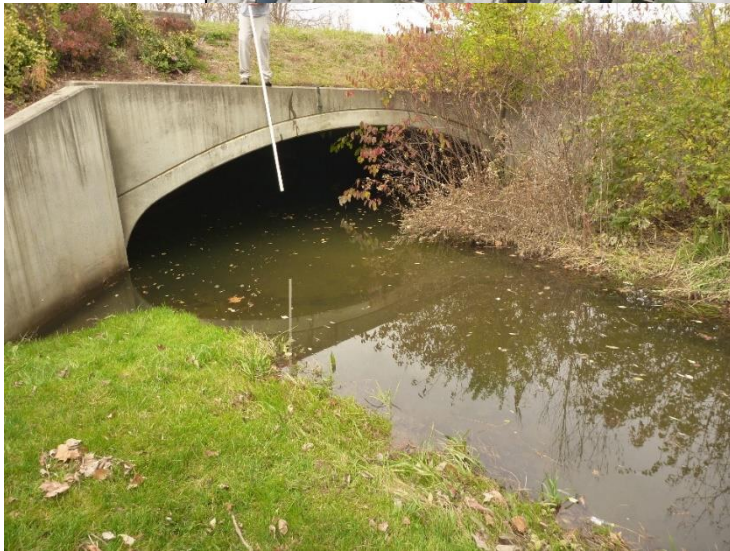
Lauren Meadows Drive Culvert
