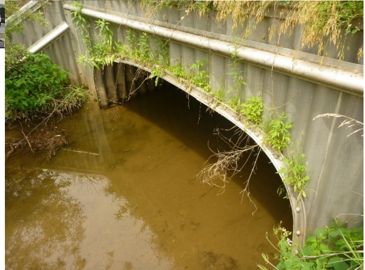
Benjamin Lane Culvert
