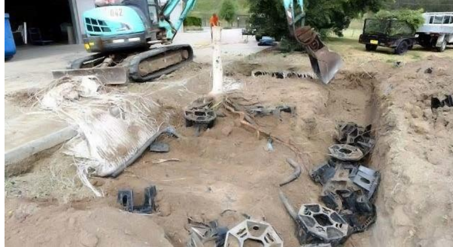
Figure 17 - the first insight into the patterns of root growth in the Stratacells is revealed once the first layer is mechanically removed. In some cases, Stratacells had to be cut away as roots had penetrated the cells.
