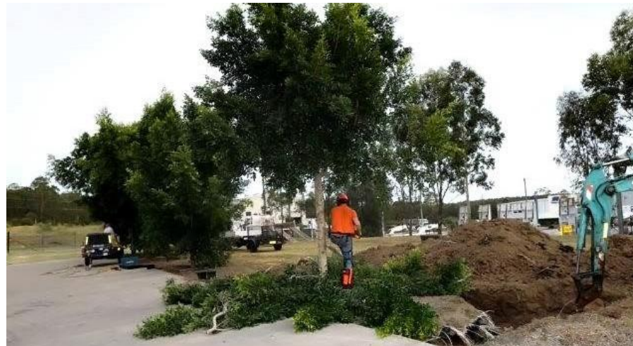
Figure 12 - removing the canopy to permit access for further work.
