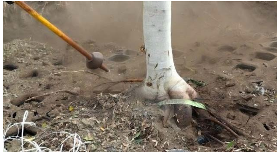
Figure 16 -the high pressure air easily exposes the first layer of Stratacells and the initial root crown.
