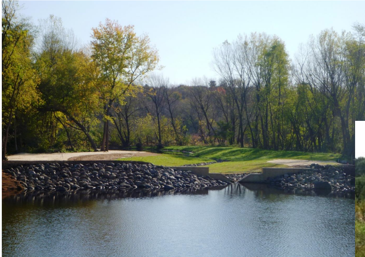
Looking downstream at the natural channel and stilling pool/wetland restoration.
